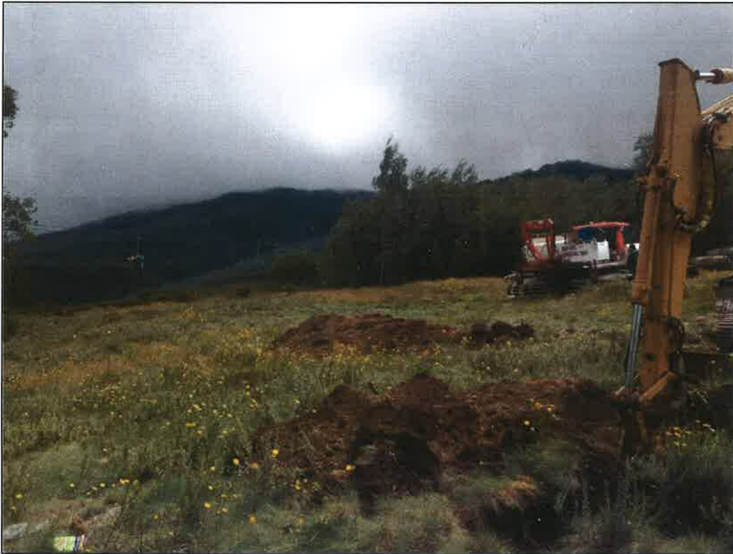
Plate 2: Looking upslope to the north west.
